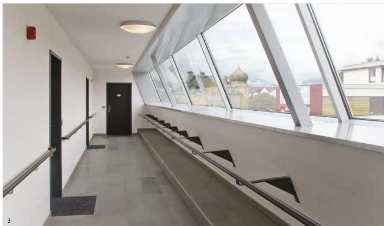
3 Entrance marking, handrail as orientation aid – Tyrol Centre for the Blind and Visually Impaired (Architekt DI Mayerhofer, architektur-ps, photo by Magdalena Possert)
