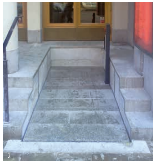
1, 2 Lifting platform integrated into stairs – Folkoperan Stockholm (photo by Guldman)
