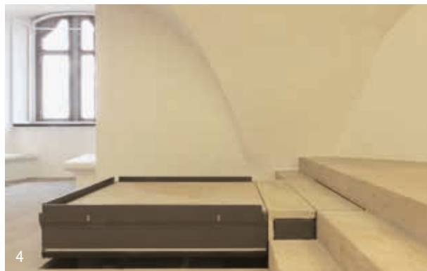
2–5 Integration of a lifting platform into a historical flight of stairs at Albrechtsburg near Meißen. As an anti-trap safety measure, the lifting platform was framed with a sensor strip to switch off the mechanism upon accidental contact (Raum und Bau GmbH, photos by Alexander Krippstädt).
