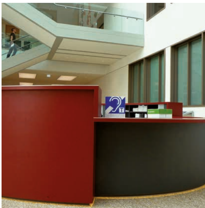
2 Information counters at various heights and audio induction loop systems – Local and Regional Court Düsseldorf (agn Niederberghaus & Partner GmbH)
