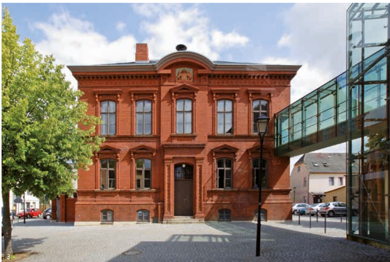
3 Outdoor lift – Former Local Court, Town Hall, Malchow (Autzen & Reimers, photo by the Heritage Conservation Office of Mecklenburg Western Pomerania, A. Bötter)
